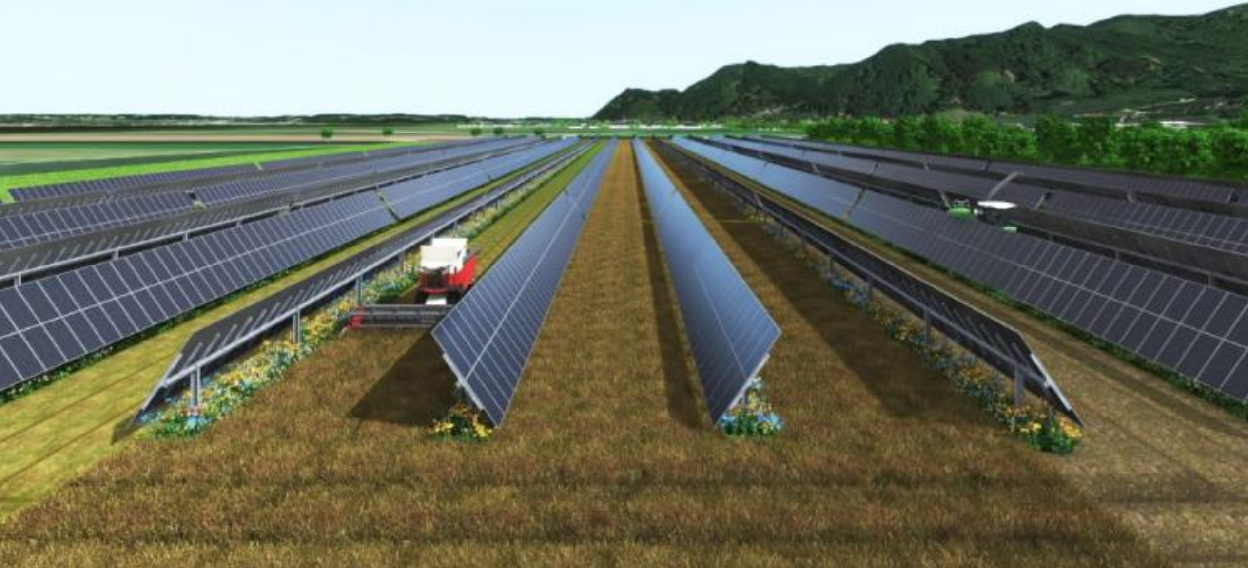
AGRI PV at Bruck/Leitha – 3 MW – single axis tracked
